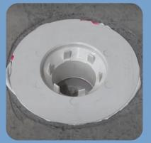
It is preferable to rebate the drainage flange into the substrate.
